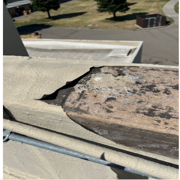
Brown Mastic/Sealant at Roof Cap
